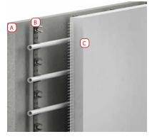
A Brick wall B Pipe-fitting track C Mortar-based plaster with plastering mesh
